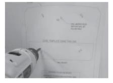
2. Drill holes for the wall anchors with 5/16" drill bit. Install anchors.
