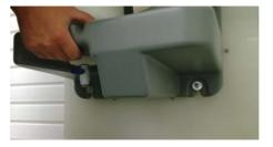
2. Hang Biocide Feeder on the two bottom screws and drill the top mounting hole locations. Remove unit from the wall and insert top two anchors. Then re-hang the unit, install top mounting screws, and tighten all screws.
