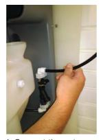
4. Connect the water supply to the inlet ball valve push-in fitting. (If you are using copper tubing, use a small section of the supplied tubing and the inline connector to connect the copper tubing to the plastic tubing. This will insure you will have a secure connection on the copper tubing away from the biocide fumes.)
