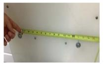
1. Drill holes for the four wall anchors with a (9/32") drill. Drill the two bottom holes 13-13 1/8" level across, insert wall anchors and thread in screws about 1/2" deep with washer on them.
